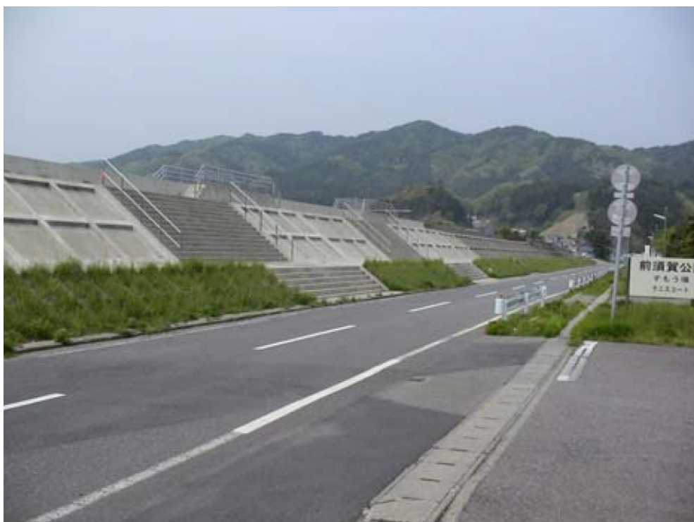
Fig. 2.1 12.8m Seawall at Funakoshi Bay in Yamada Town (Source: Takahashi, Tsunami Disaster Mitigation in Japan, 2012)
