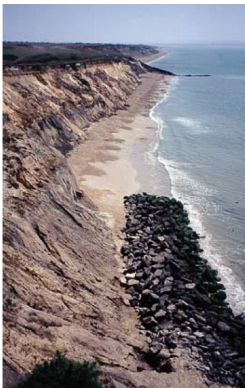
Fig. 3.11 Rock armour protection of cliff base in Normandy. (Redrawn from: Pranzini E., and Williams A., “Coastal Erosion and Protection in Europe”, 2013)
