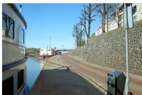
Fig. 3.3 a) two-level quay wall ( Source: Voorendt, 2014 )
