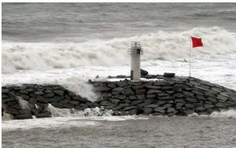
Fig. 3.13 A Rubble Mound Breakwater in the Black Sea Coast of Turkey
