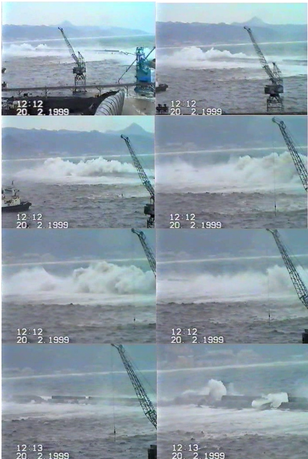
Fig. 3.14a A collage of scenes from Giresun Port under wave attack in the Black Sea Coast of Turkey
