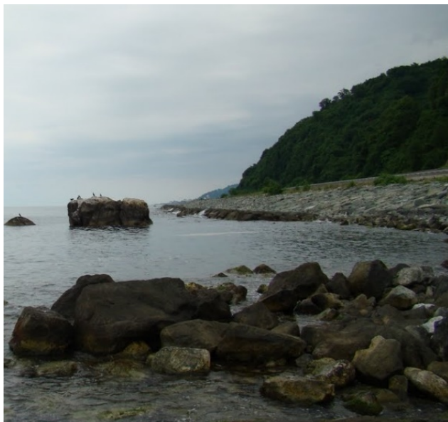
Fig. 3.12 Coastal Roadside Rubble Mound Revetment in Black Sea
