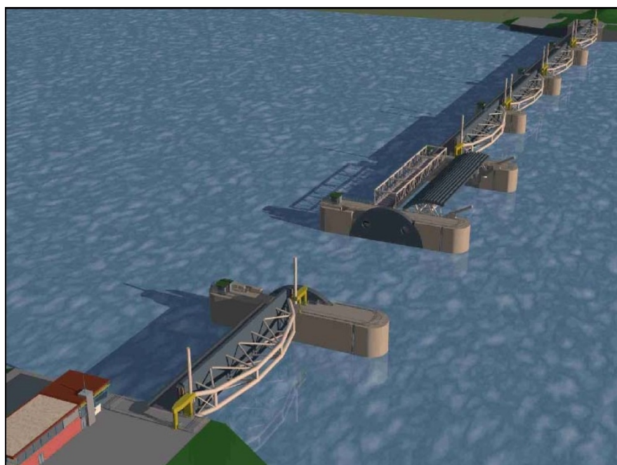
Fig. 3.8 Emssperrwerk (storm surge protection / storage function). (Source: H. Oumeraci, “Coastal Engineering” Lecture Notes, TU-BS)
