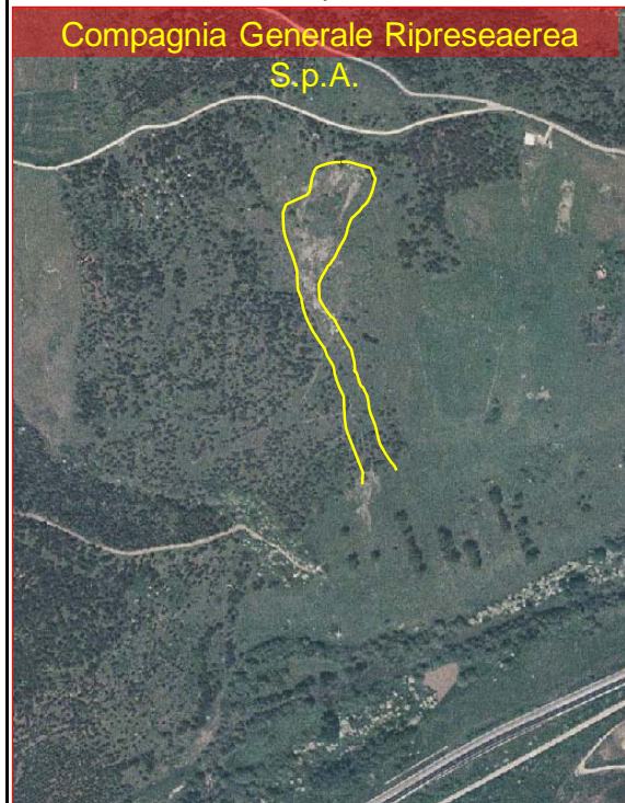
Figure1: Aerial photo of Masseria Marino landslide
