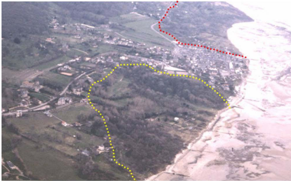
Aerial view to the West on the Villerville-Cricqueboeuf landslides (1988)
