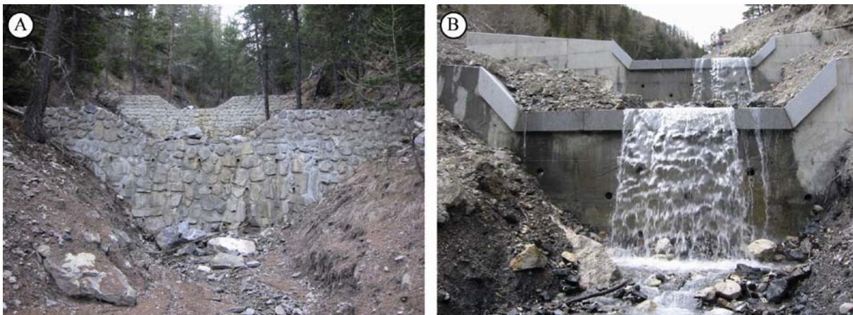
Figure 4.2 The two main types of check dams in the Faucon torrent: (A) photograph of a masonry check dam (Champerousse torrent); (A) photograph of a concrete check dam (Faucon torrent).
