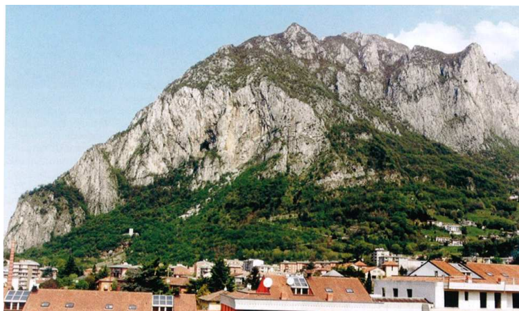
Figure 3-39. General procedure adopted for the Landslides susceptibility Map South view of the Mt. San Martino – Medale cliffs
