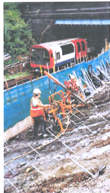
Restricted access soil nailing
