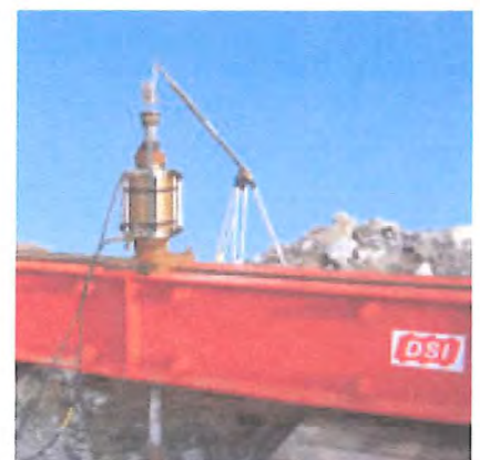
Heavy duty spreader beam for micropile tension test
