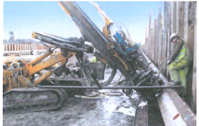
4m long T76 bars for 32 m deep anchors, sheet pile tie-back
