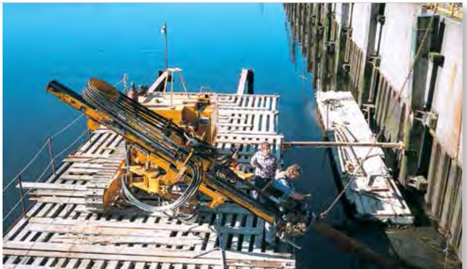
Additional anchors for a sheet pile wall, HPA, Port of Hamburg
