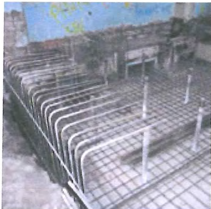
Base slab reinforcement using micropiles
