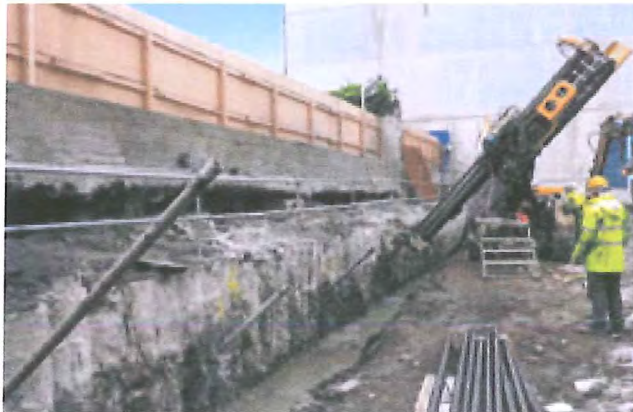
Drilling through a secant piled wall
