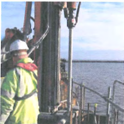
Grout injection behind sheet piles
