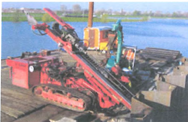
Hollow bar drilling from a floating barge for sheet pile tie back
