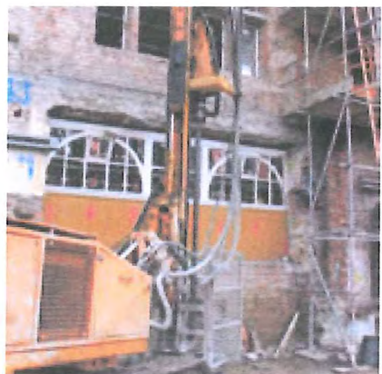
Micropiles for retained facade frame bases
