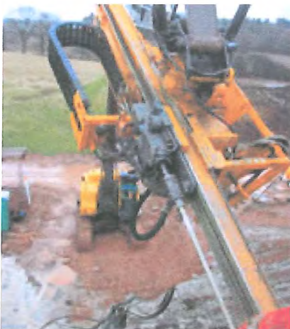
Drilling with long reach excavator
