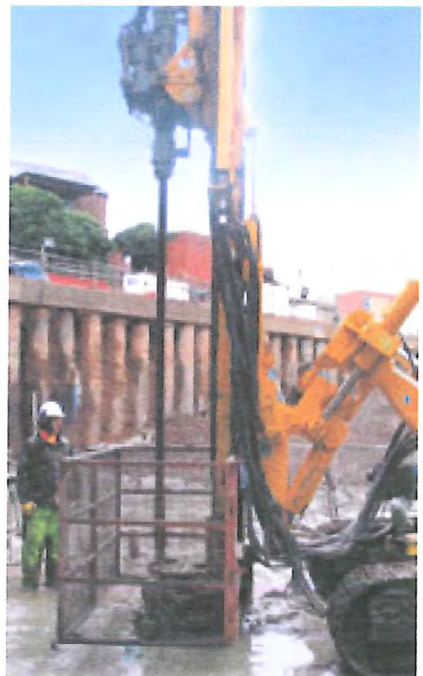
Long stroke drill boom for deep micropiles
