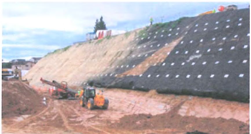
DYWI® Drill Hollow Bar soil nails with reinforced geogrid facing
