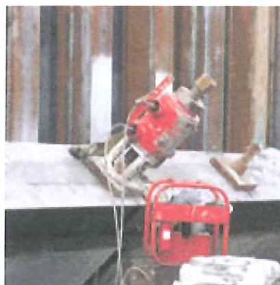
1,500kN jack for T76 temporary anchors
