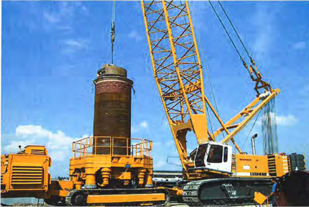
RDM-M 2000 in operation
