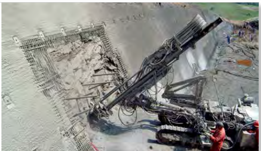
Remainder of embankment stabilised with soil nailing
