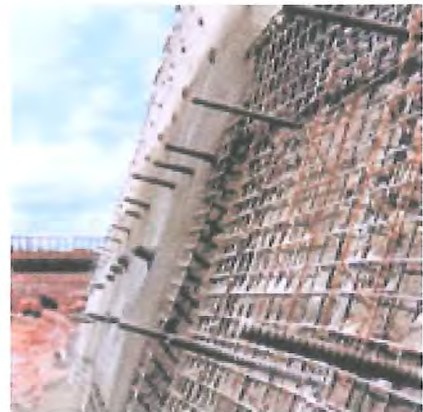
Grouted soil nails on shotcrete face
