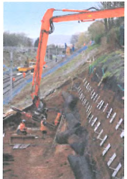
Long reach excavator for restricted access drilling
