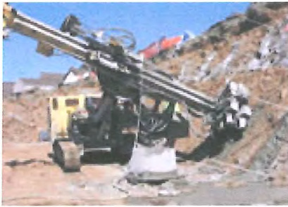
Crawler mounted drill boom for simultaneous drill & grout soil nails
