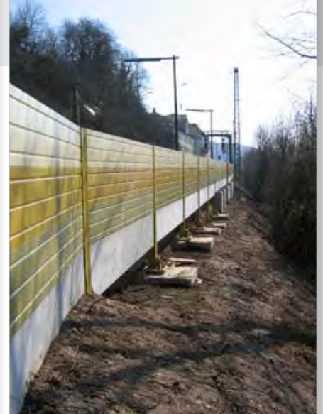
Foundation to noise barrier adjacent to Karlsruhe–Freiburg railway line, south-west Germany
